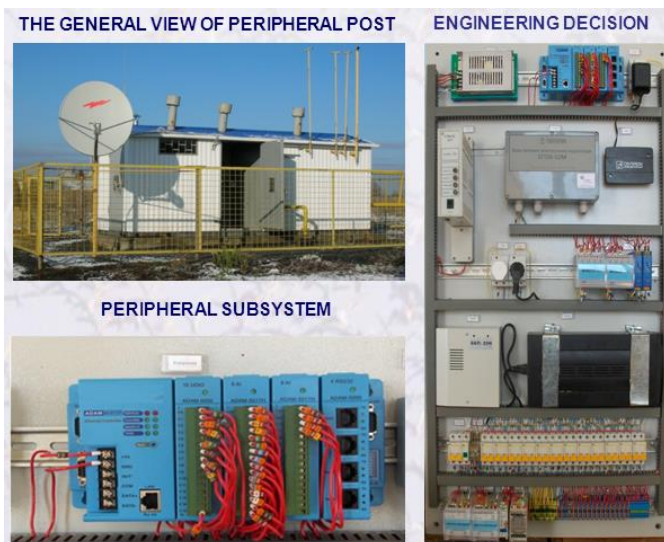
Figure 7. The Complex of supporting technogenic safety on the objects of oil & gas distribution
