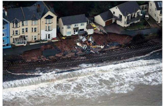
Figure 2. The breach in the sea wall near King Harry's Walk at Dawlish, Devon, on 7 February 2014
